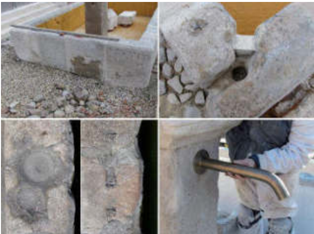
Figure 5.- Restoration details: substituting cement for limestone and pylon waterproofing; discovery of the primitive spillway corner; conservation and protection of the original remains; new sewers made of brass as per the primal design.
