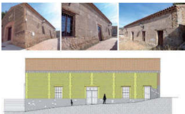
Figure 1.- “Salón del Cuco” construction placed in Burbáguena made with columns of pure gypsum.
