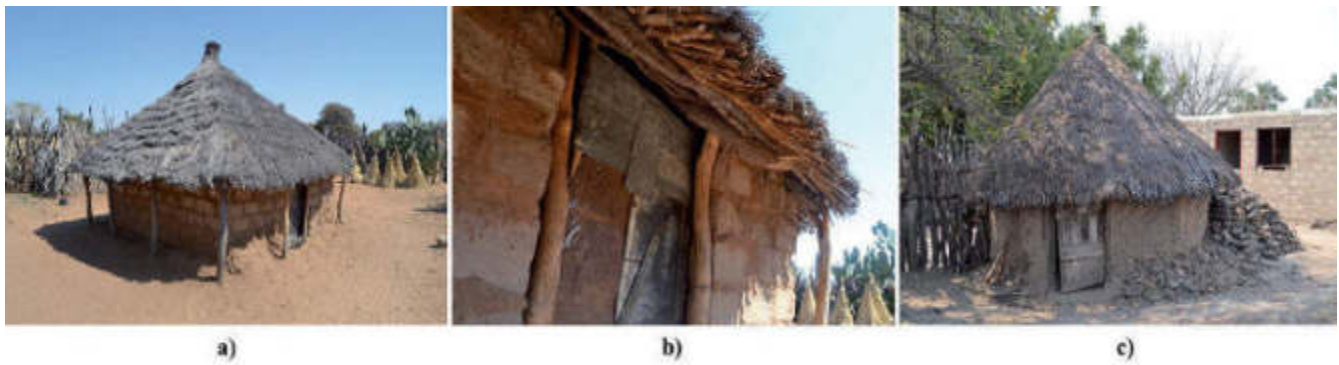
Figure 5.- a) One example of an adobe hut within the case study homestead. b) Detail of the connection between adobe masonry walls and the thatch roofs. c) An example of a vernacular structure in an advanced state of degradation due to the increasing abandonment of vernacular constructive techniques to the detriment of imported building technologies and materials.
