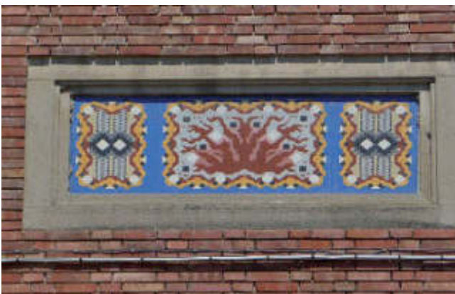
Figure 3.- The mosaic of the former stable calibration
