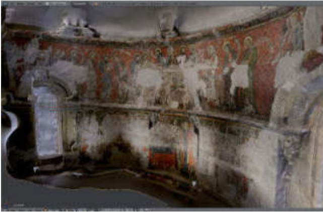
Figure 3.- Three-dimensional view of the mural paints of the Collegiate church of Daroca made by convergent photogrammetry.
