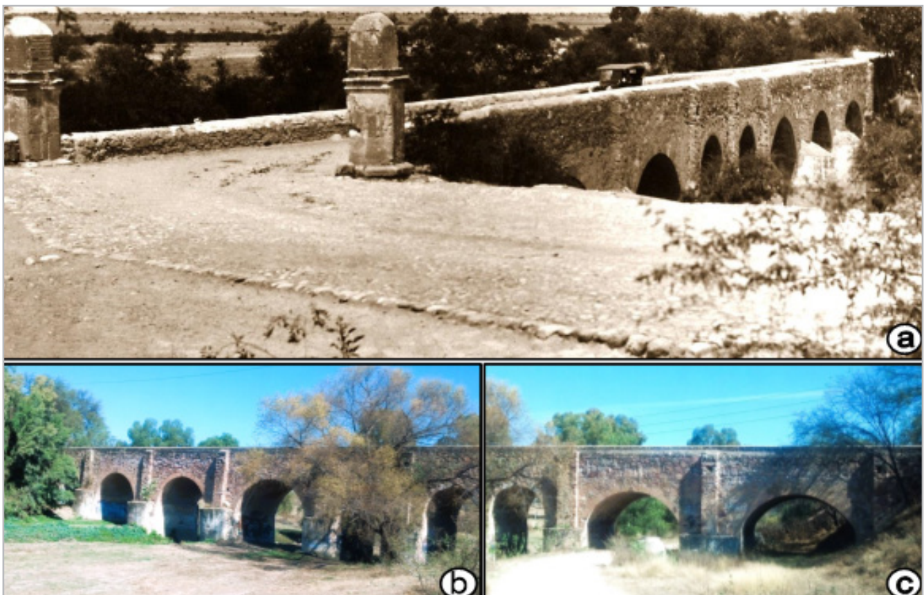
Figure 2.- Old and recent images of the San Ignacio Bridge. a) Photo from the beginning of the XX century. Original boulder paving and the approach with a different direction than the current one. b) Arcs from axis A to H are shown. c) Arcs from axis G to J are shown [Figure 4].
