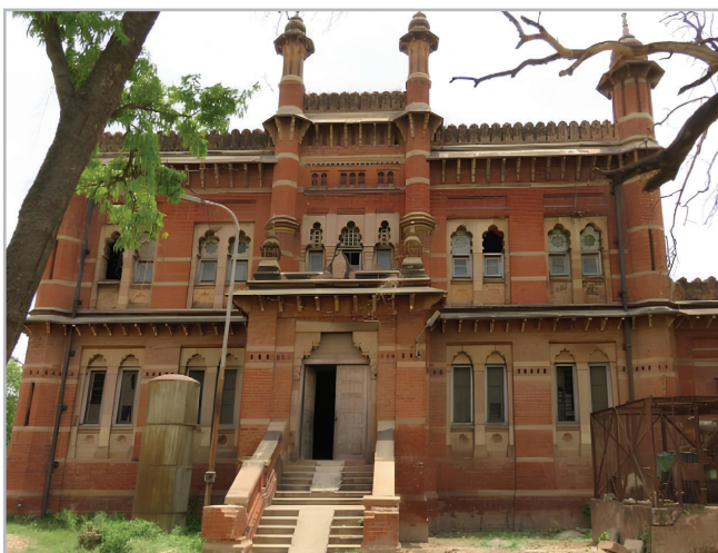
Figure 4.- The purification building of Bhelupura Waterworks in Varanasi. (Photo by author 2017)
