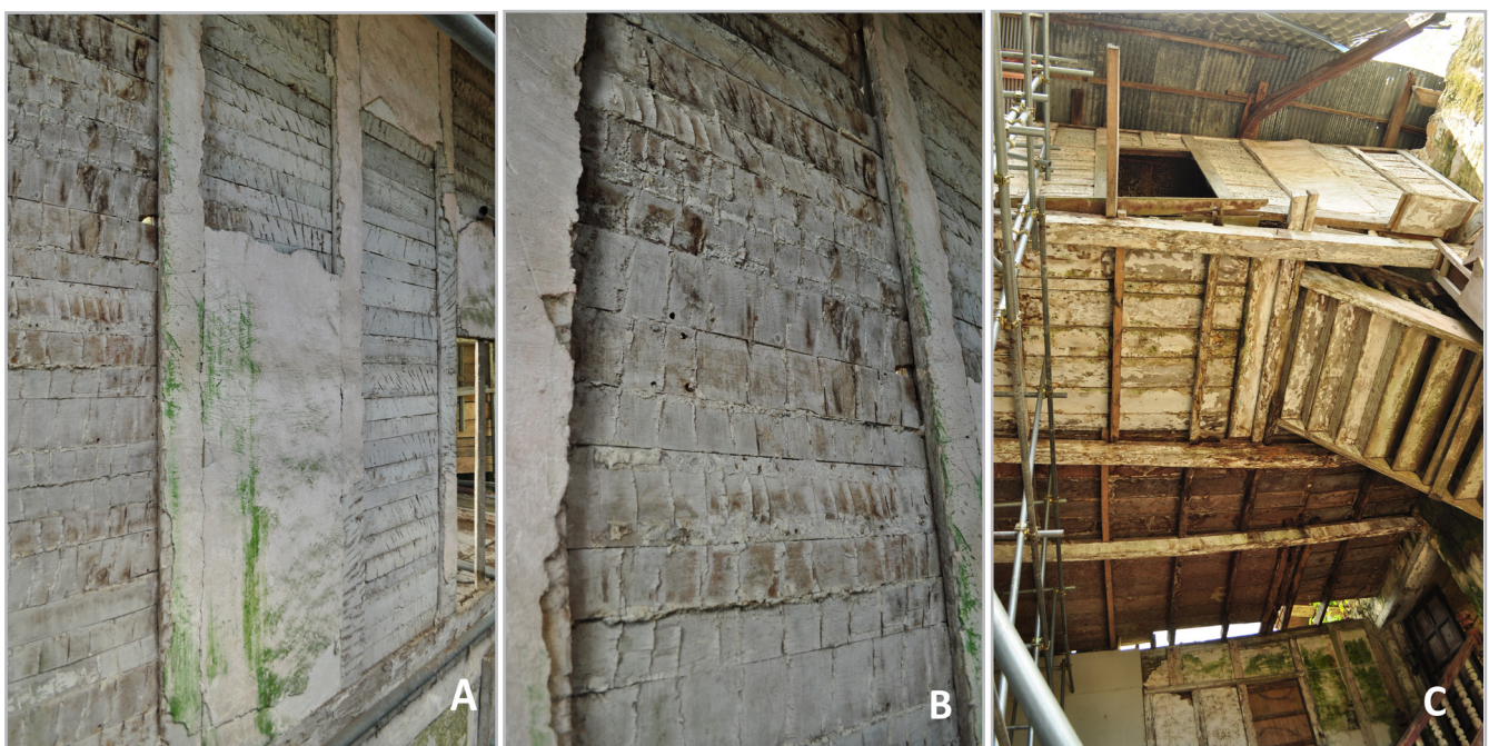
Figure 2.- Wall partition using the tabique Pampango (wattle-and-daub) technique. (A) and (B) shows the daub collection site with the exposed wattle frame. (C) is the view of the wall partition inside the 19 th century Loboc church convent
